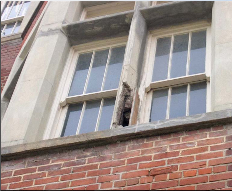
Examples of Precast Concrete Deterioration
